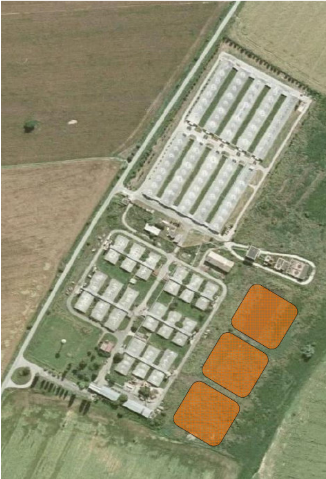
Annex 01.3: Farm after renovation, Photo and sketch of overview
